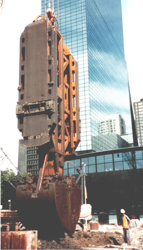
Fig. 2 Clamshell excavator for the foundation walls
