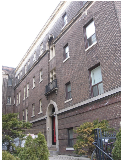
Courtyard wall (south)
