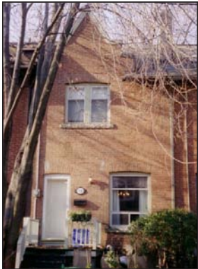
No. 64-70, designed by Architect E.G. or S. Wilson
