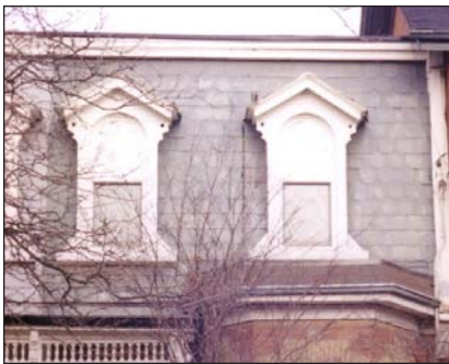
surviving decorative slate roofing
