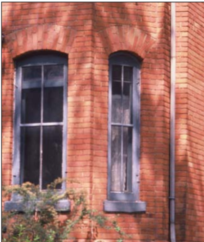
restored Victorian wood windows with wood storms, Cabbagetown
