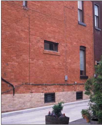
restored masonry, Laurier Avenue, Cabbagetown
