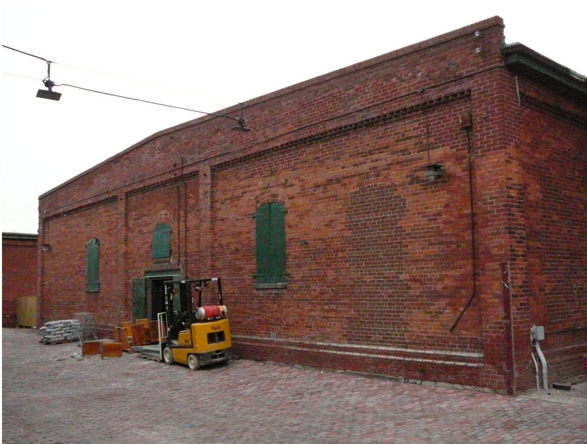
Rack House G (Building 64), Tank House Lane/North Elevation
