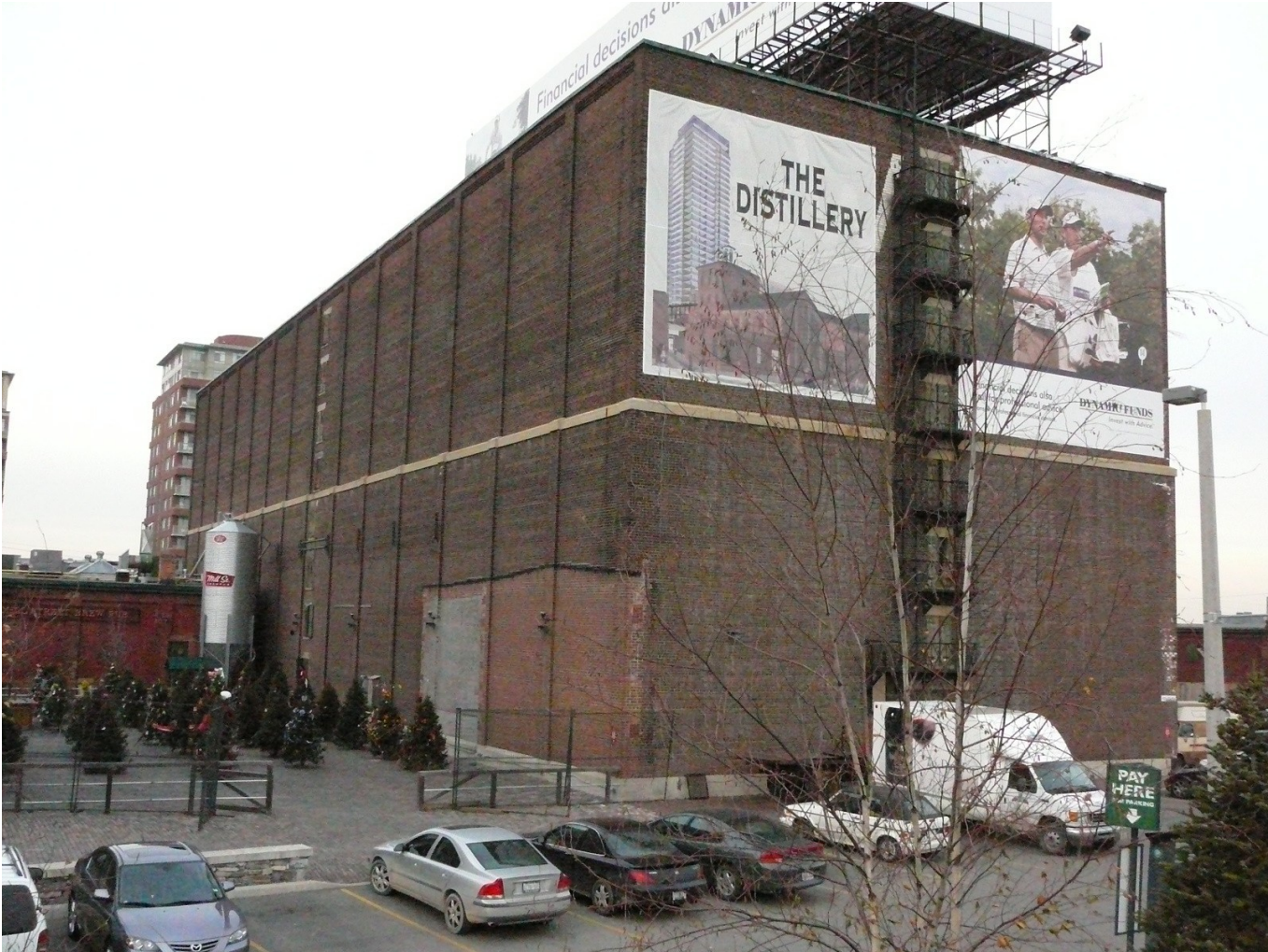
Rack House M (Building 75) South Elevation
