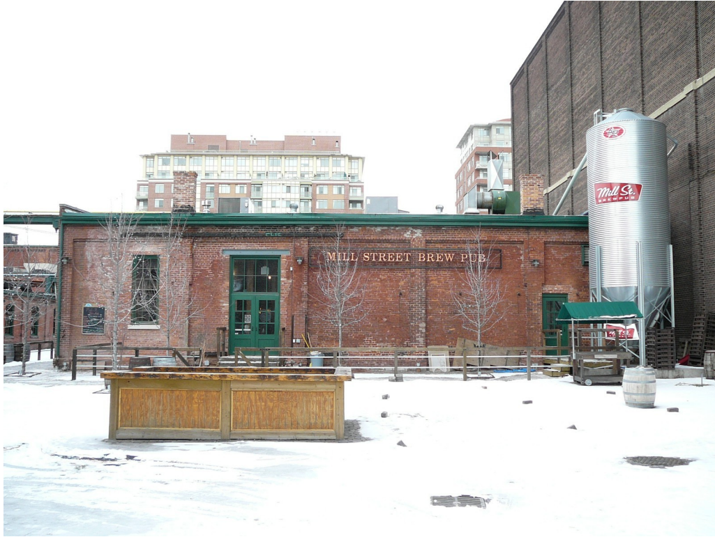
Paint Shop (Building 63), South Elevation
