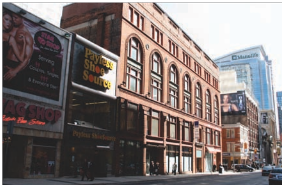
Before: inconsistent intensity of signage and discontinuity in the street wall
