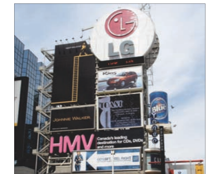
Media Tower installed on building
