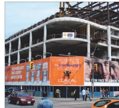
Signage applied to temporary hoarding
