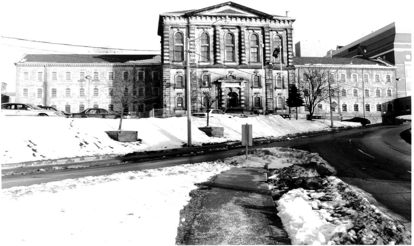
Schedule "C" Photograph – City Heritage Easement Agreement View of the principal (south) façade showing the 4-storey centre block flanked by the 3 ½-storey west (left) and east (right) wings.
