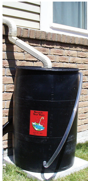
Downspout disconnection rain barrels reduce storm sewer overload and provide water for lawns and gardens
