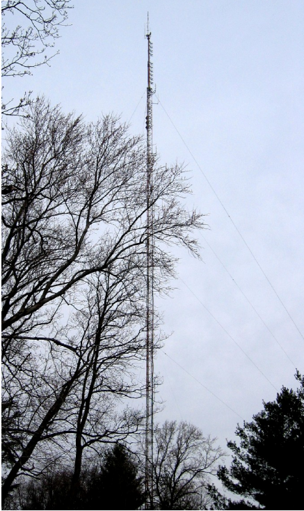
Guyed Tower (supported by guy wires)
