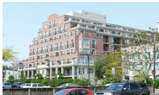
Figure 7.9 Through the use of materials, this building has a distinctive base, middle and top. The mechanical penthouse is also incorporated into the architectural design.
