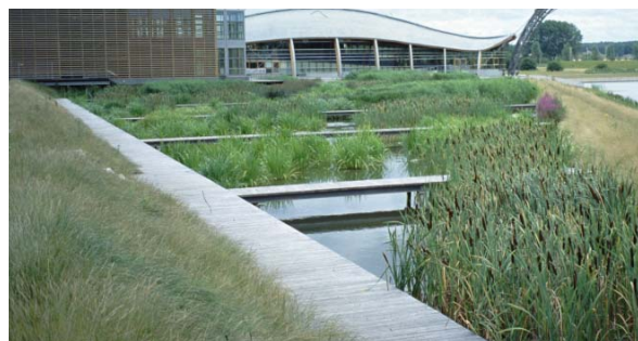
Stormwater Management Pond
