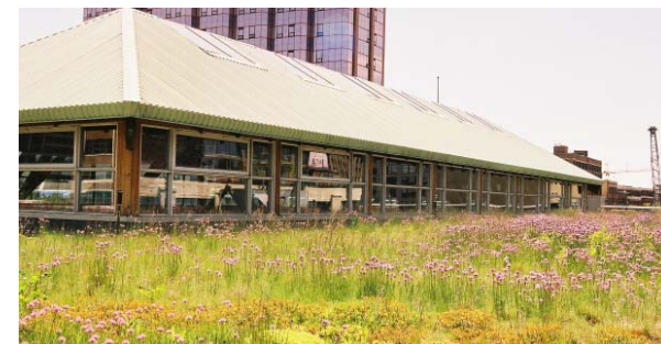
Green Roof, Toronto
