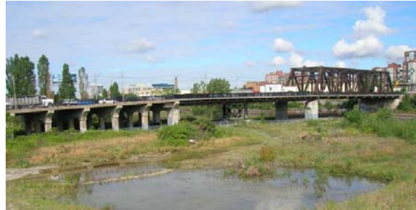
Bathurst Bridge looking northwest
