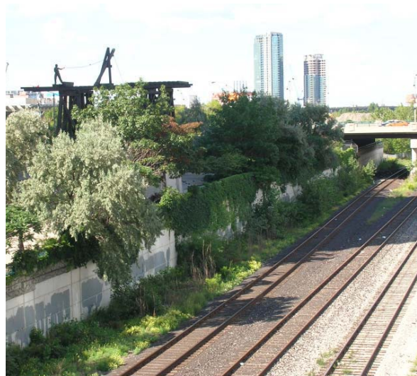
Existing retaining wall, south side at Spadina Avenue
