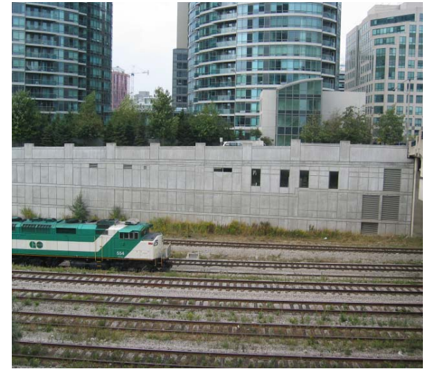
Existing retaining wall, north side at Spadina Avenue
