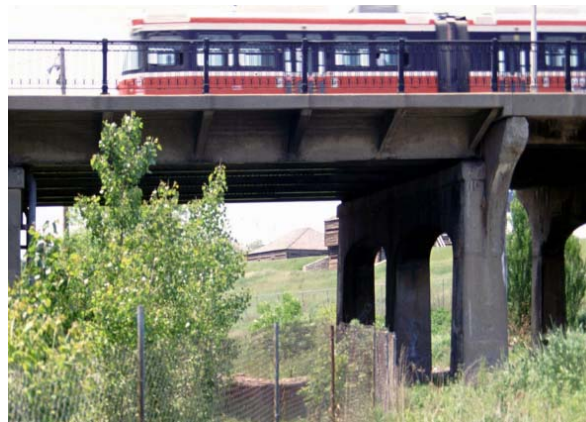
Under the existing Bathurst Bridge
