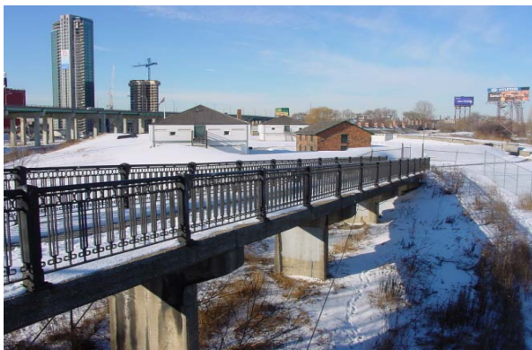
Existing Bathurst Street Pedestrian Bridge
