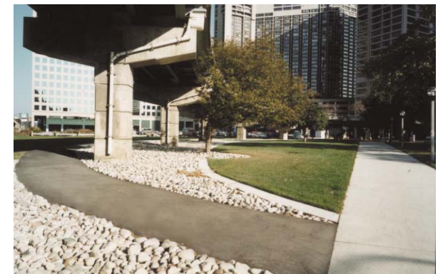
Hard landscape treatment under the York Street exit ramp
