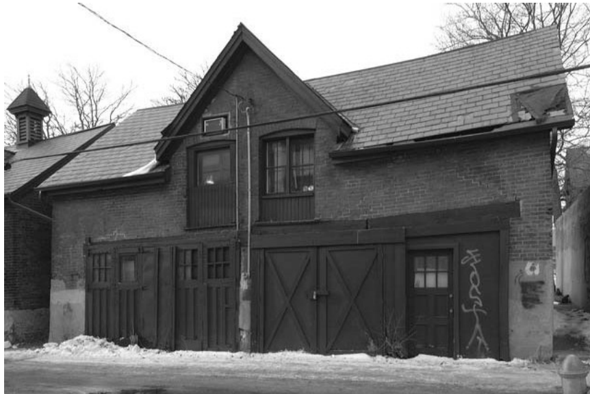
North Coach House, showing the east elevation on bpNichol Lane
