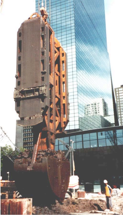
Fig. 2 Clamshell excavator for the foundation walls
