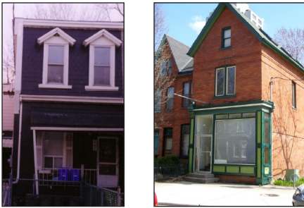
(left) No. 165, builder Frederick J. Macdonald, first group of houses 1886
