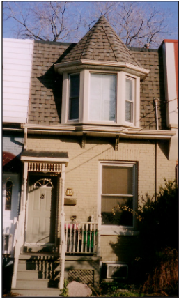
workers cottage Designed by E.J. Lennox
