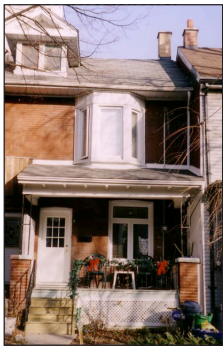
No. 57 Tiverton, carpenter William Hodgkinson
