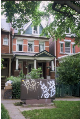
transformer on Brunswick Avenue
