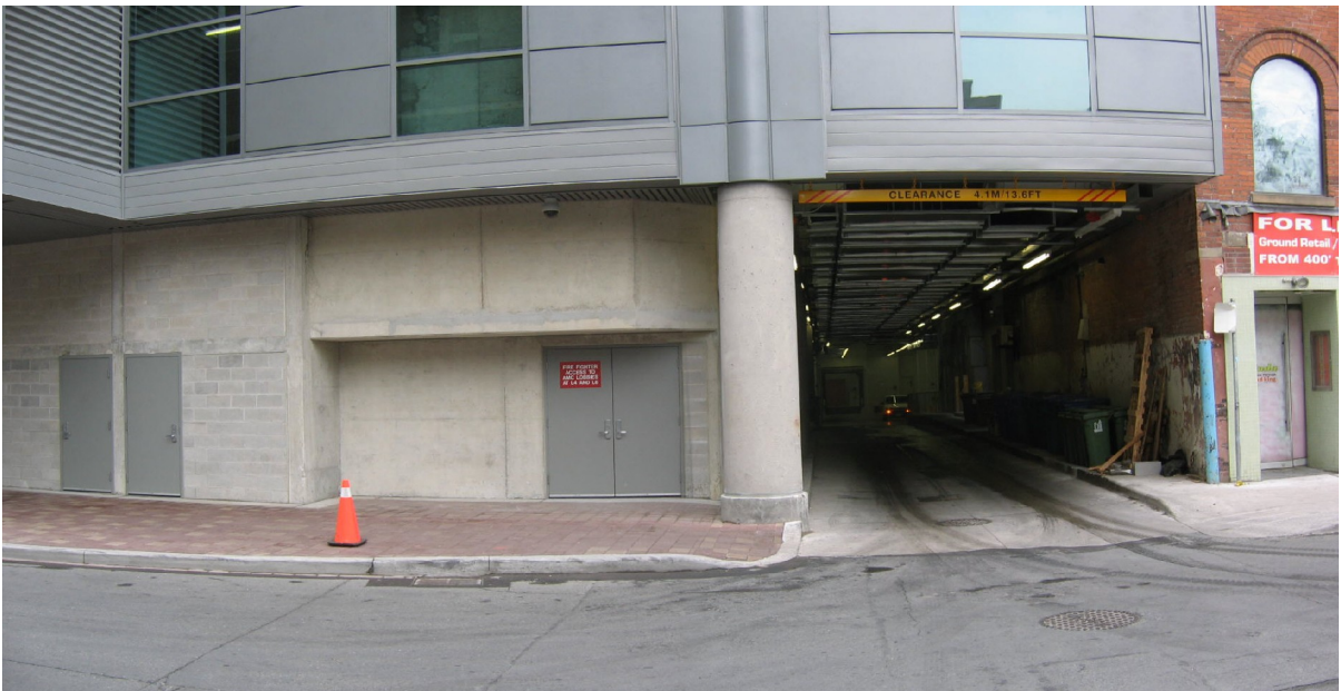
Proposed location of Ryerson Gateway Pole as indicated by the pylon - South side of Gould Street. Shipping/receiving driveway for Toronto Life Square is shown on the right.
