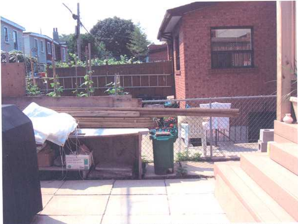
Photograph illustrates the fence along the south side of the property line, adjacent to the neighbouring property at 143 Bellwoods Avenue. The fence is 1.12m in height and is approximately 7.60m in length.
