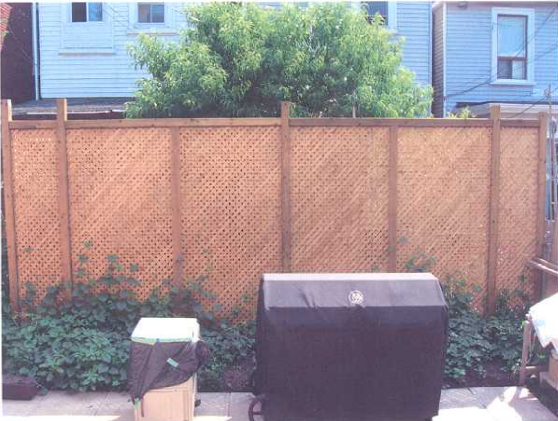
Photograph illustrates the fence along the east side of the property line, adjacent to the neighbouring property at 148 Bellwoods Avenue. The fence is 2.81m in height and 6.40m in width.
