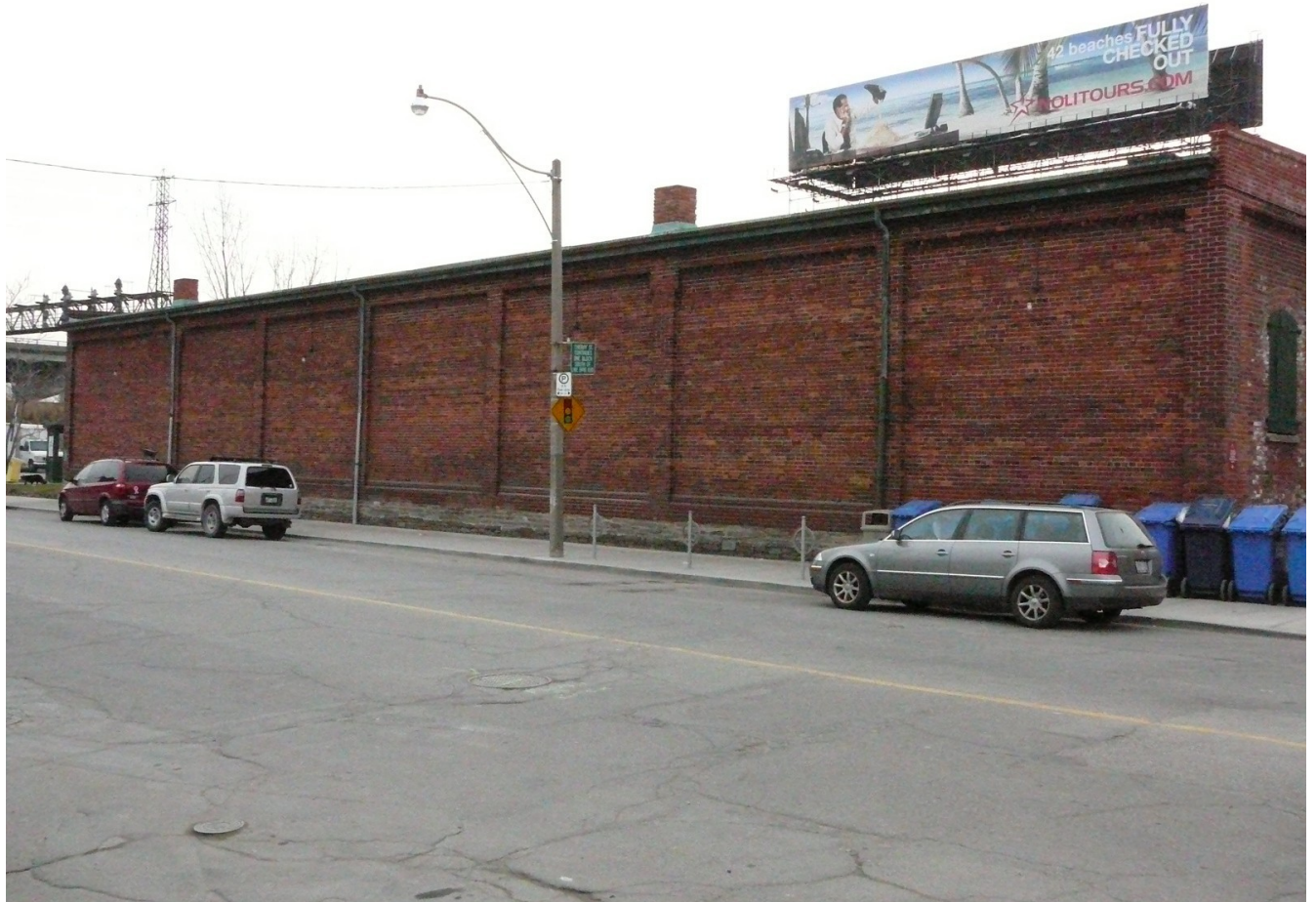
Rack House J (Building 65), Cherry Street/East Elevation
