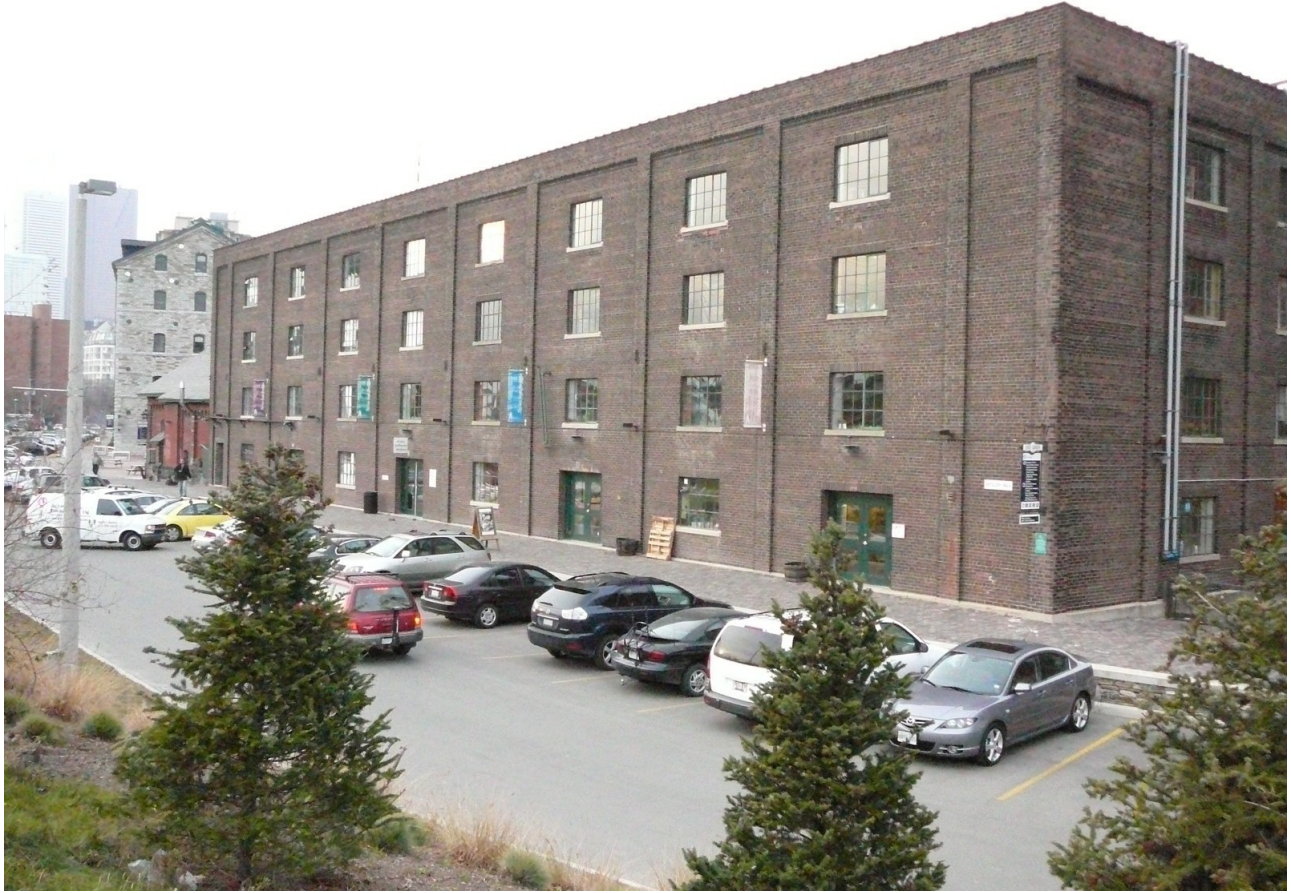
Case Goods Warehouse (Building 74), South Elevation
