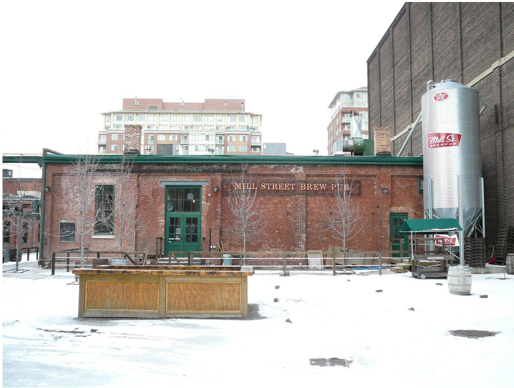
Paint Shop (Building 63), South Elevation
