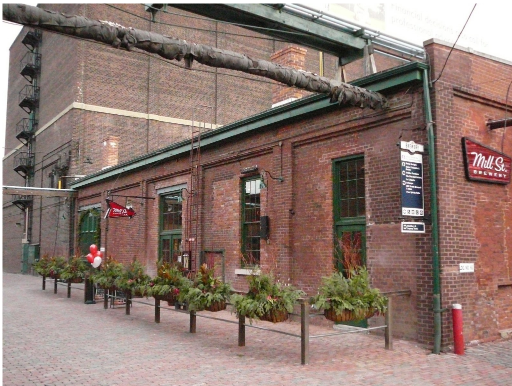
Paint Shop (Building 63), North Elevation
