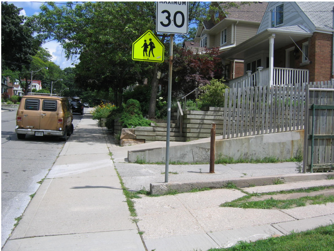
Looking East along the Glen Ames Road rear of 24 Williamson Road July 24, 2008
