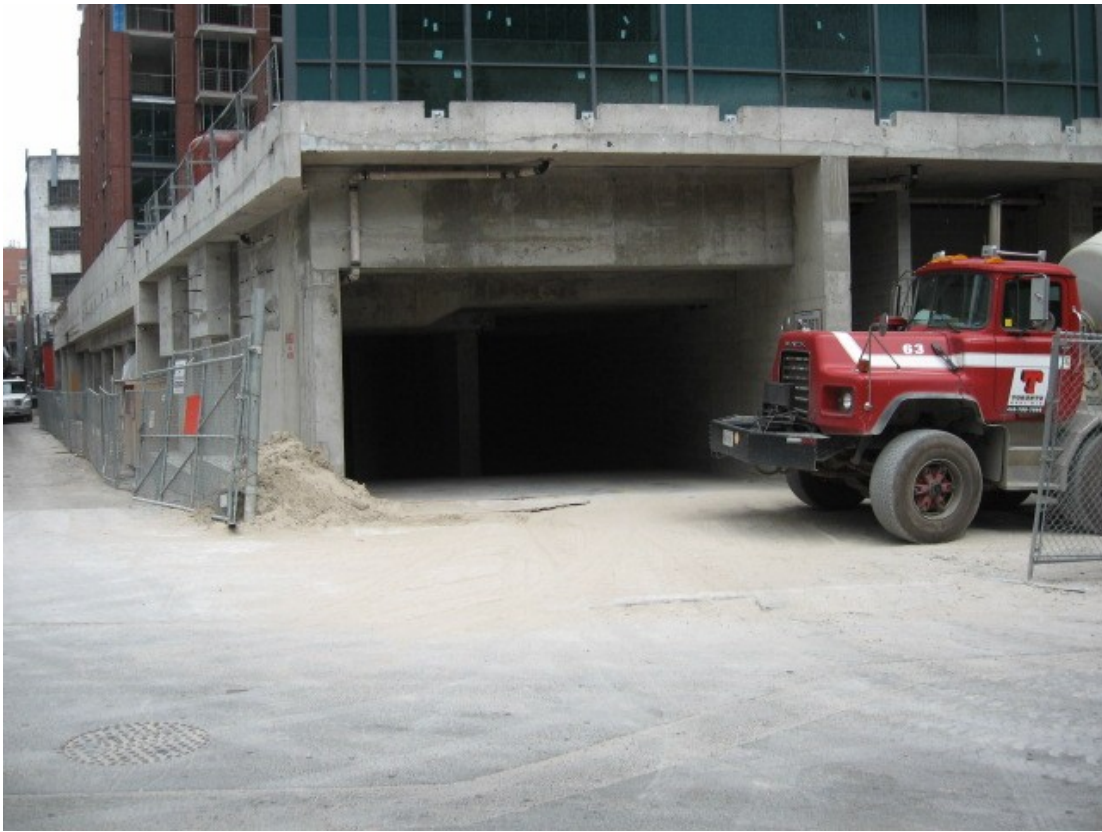
38 The Esplanade and 1 Scott Street – Garage Entrance on Scott Street – July 8, 2008
