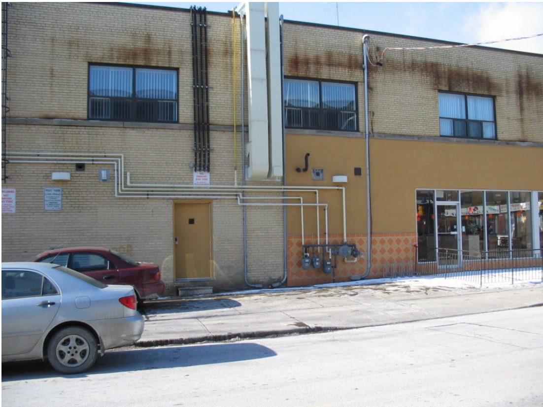
1193 Bloor Street West, Brock Avenue flank – January 25, 2008
