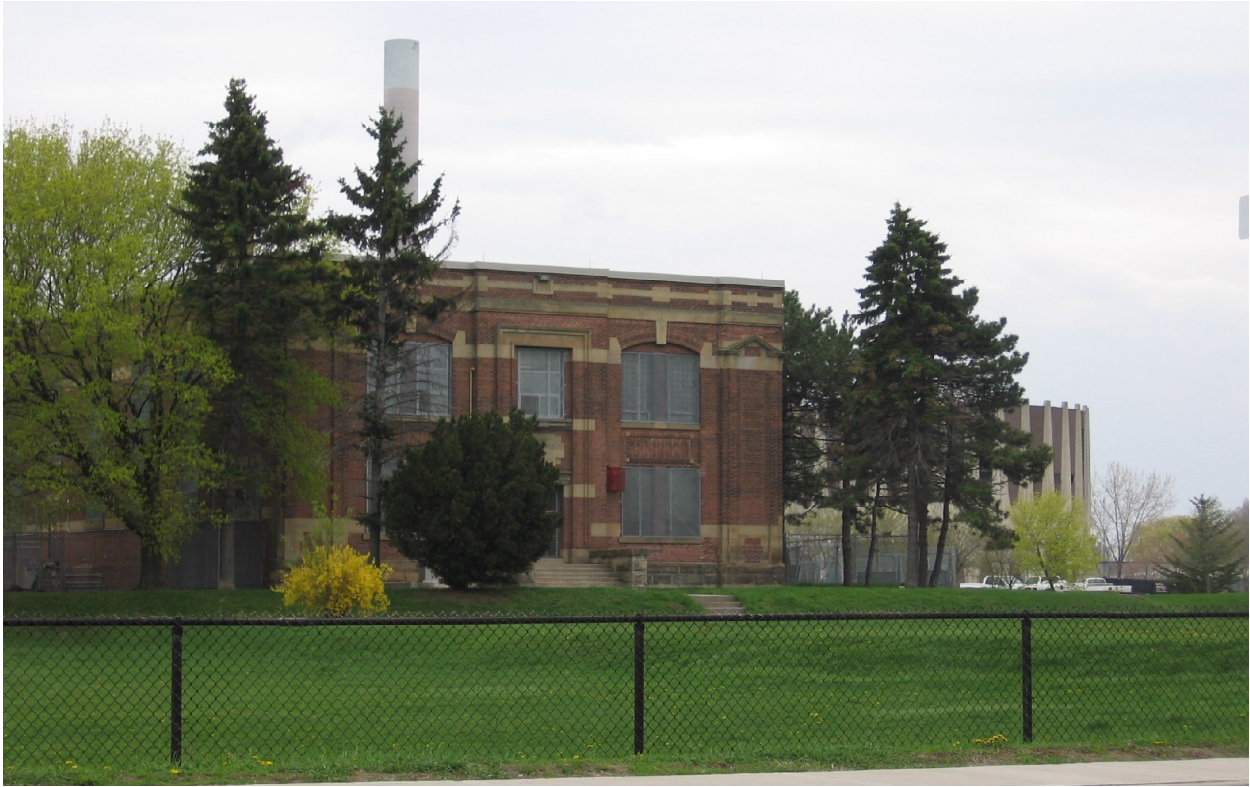
1911 (left) and 1971 (right) Pumping Stations viewed from Eastern Avenue
