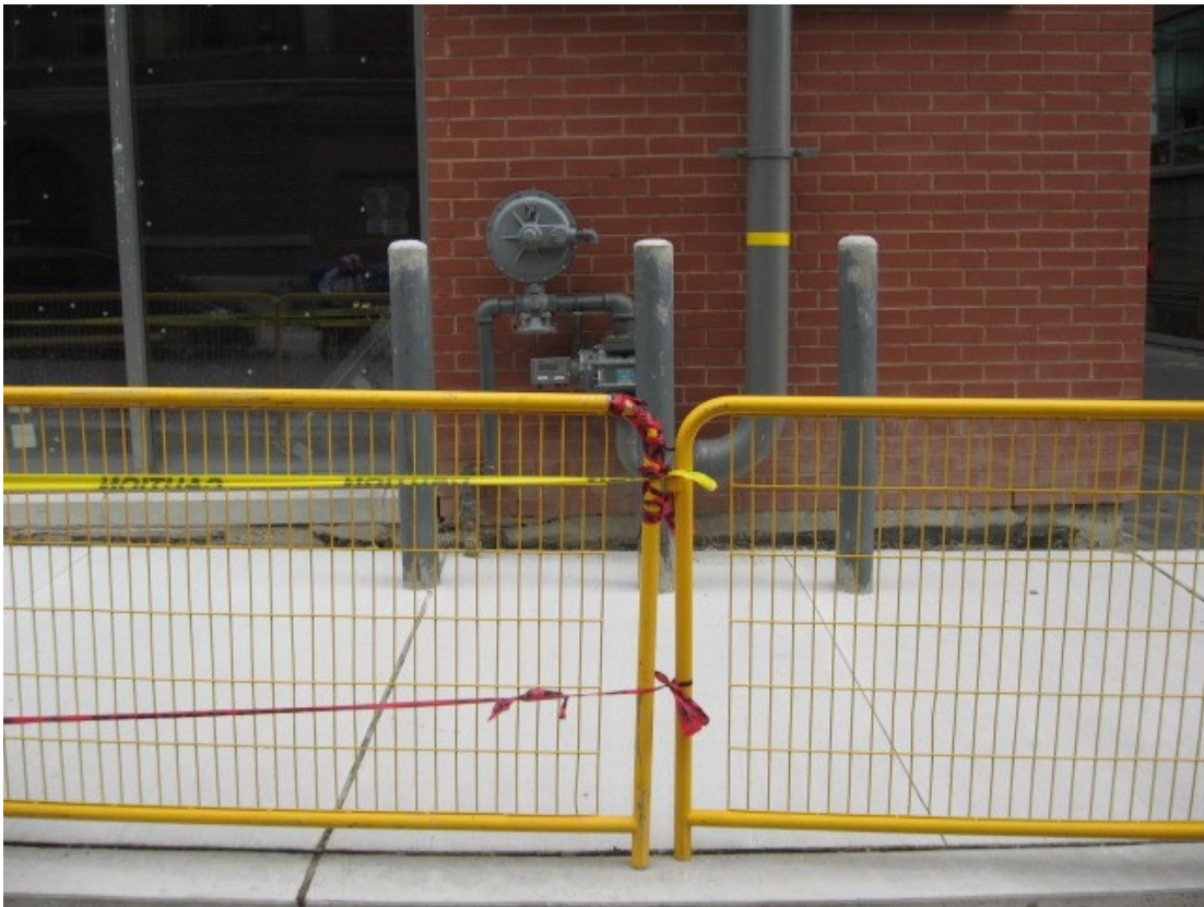
311 Adelaide Street East – Frederick Street flank September 15, 2008
