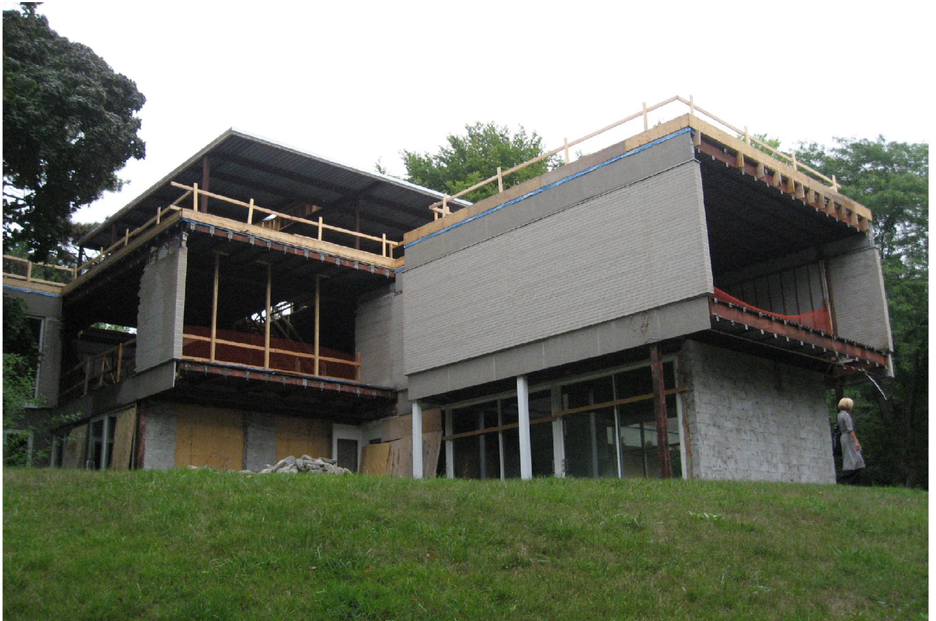
Figure 4a: VIEW OF RAVINE SIDE: photo taken in Fall 2007
