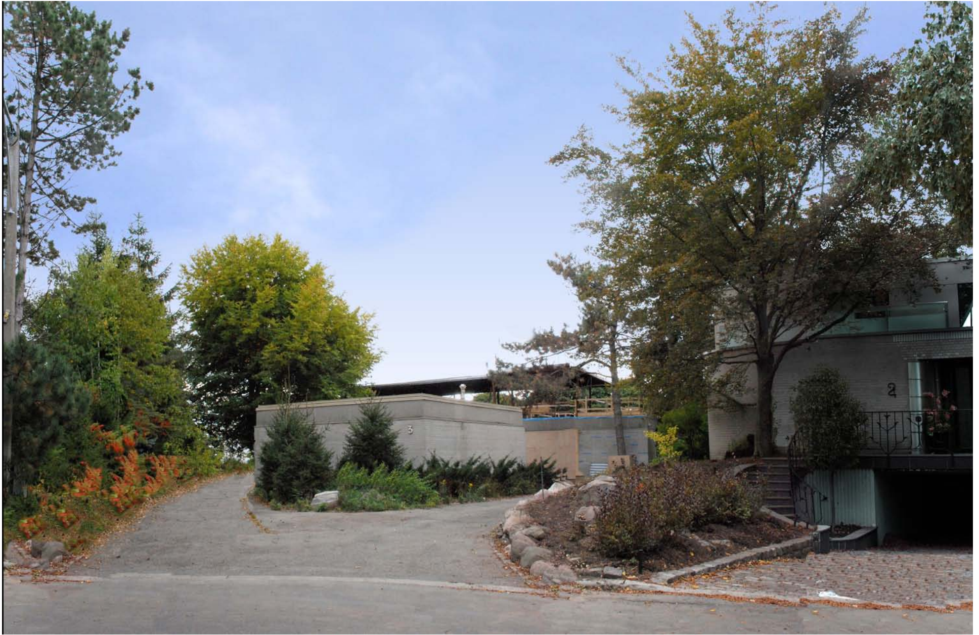
3 OLD GEORGE PLACE VIEW FROM STREET SIDE: EXISTING CONDITION
