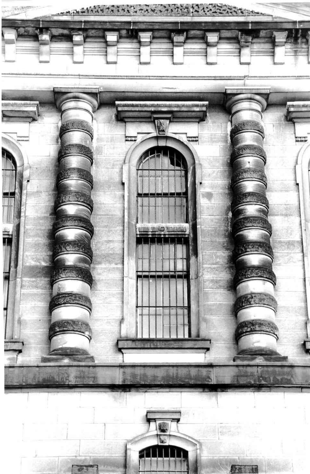
Schedule "C" Photograph – City Heritage Easement Agreement Detailed view of the centre block, showing one of the two-storey round-arched window openings with stone detailing and iron bars in the upper floors of the south façade.
