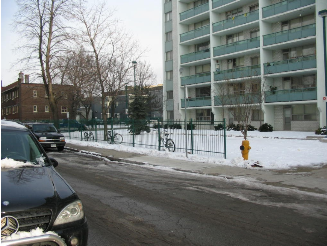
730 Dovercourt Road – January 4, 2008
