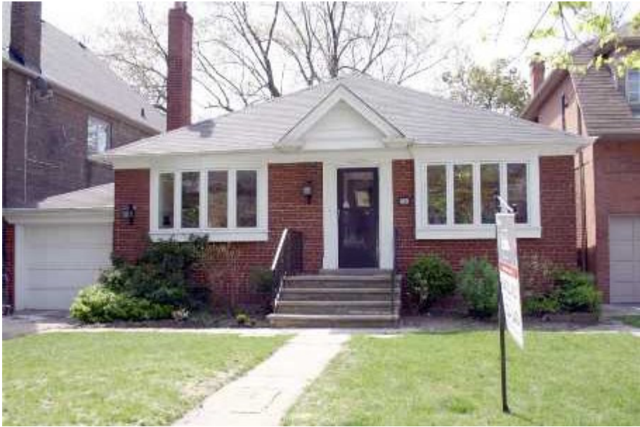
19 Whitehall Road – un-rated structure
