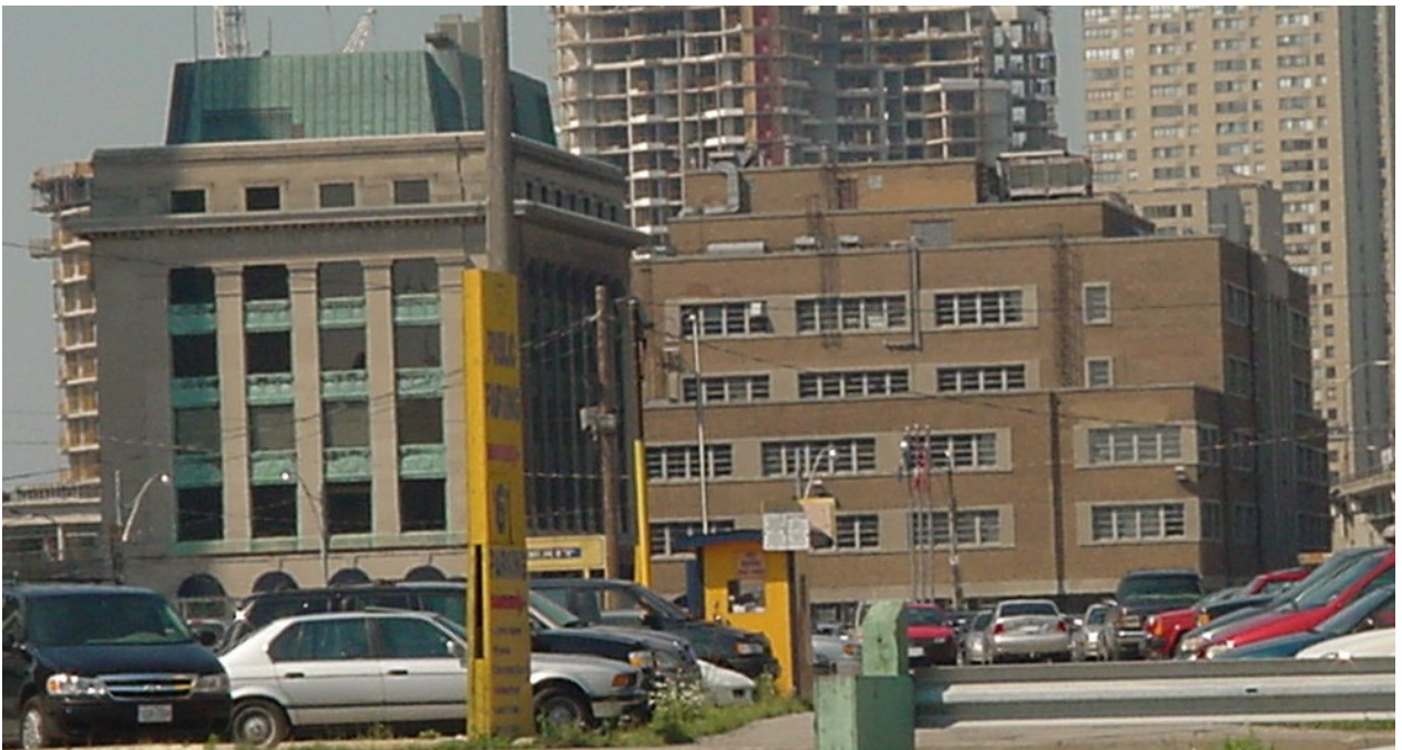
View looking west from Bay Street to York Street, and showing the Toronto Harbour Commission Building at 60 Harbour Street (left) and the Workmen's Compensation Board Building at 90 Harbour Street (right)
