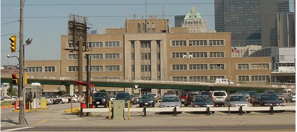
South façade of 90 Harbour Street
