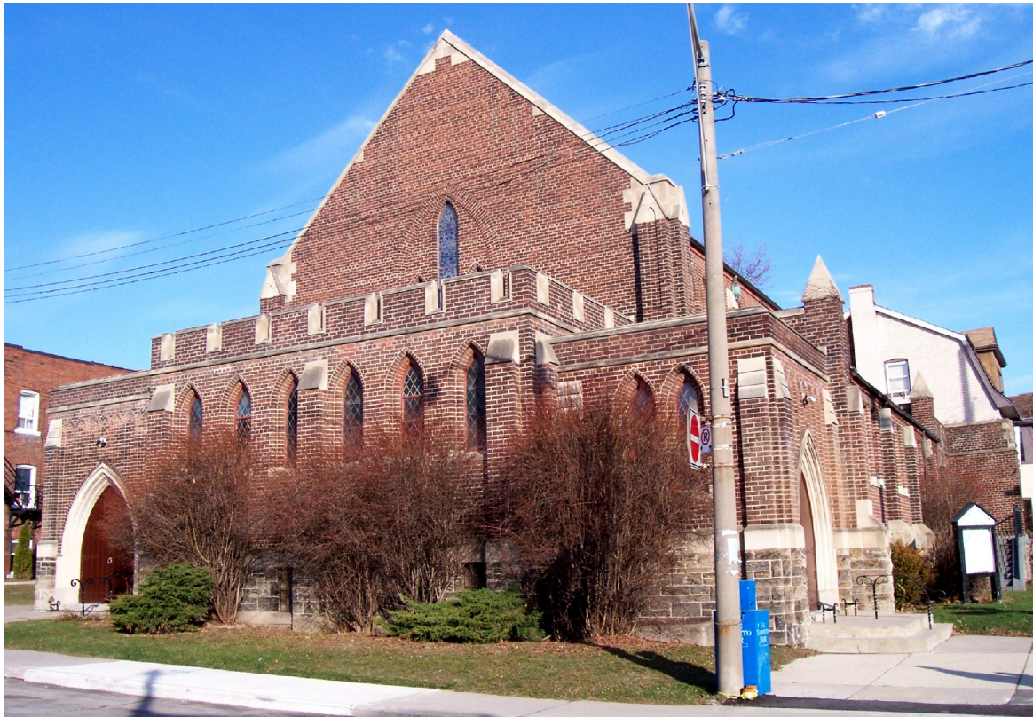
Principal (west) façade on Wychwood Avenue (left) and south elevation on St. Clair Avenue West (right)
