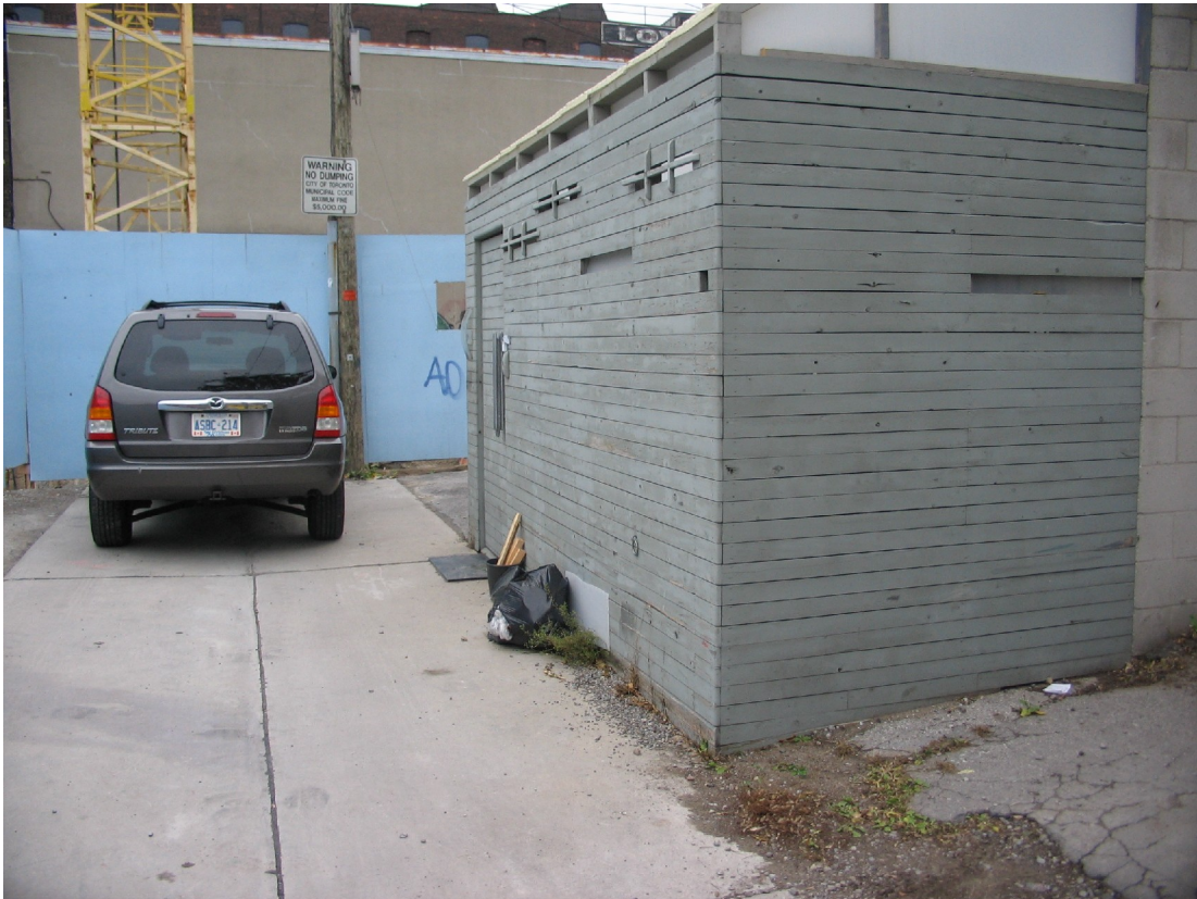
Rear of 451 Adelaide Street West November 14, 2006
