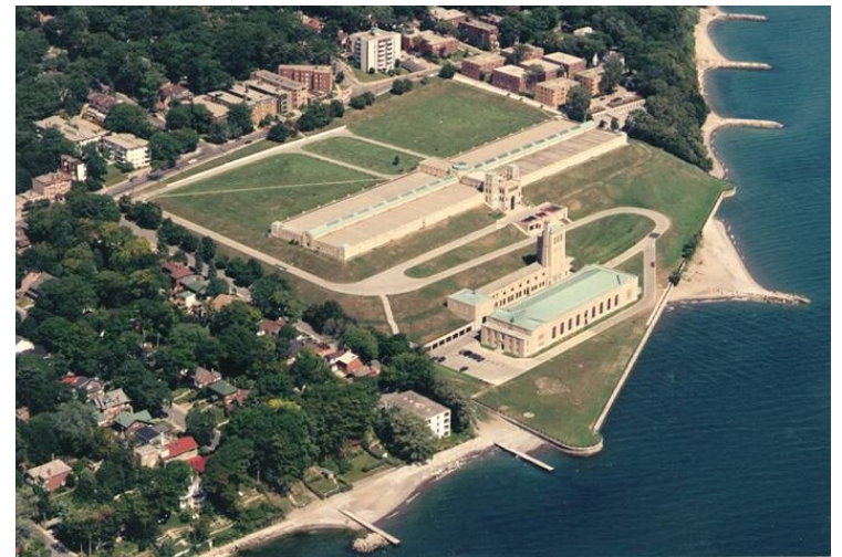
R.C. Harris Water Treatment Plant
