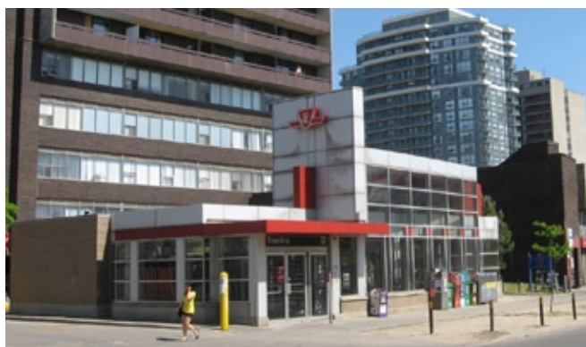
TTC entrance at Walmer Road
