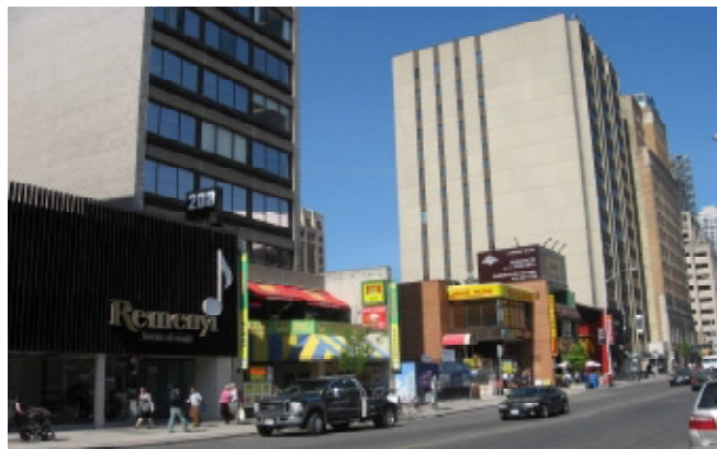
North side of Bloor Street, looking east toward Avenue Road
