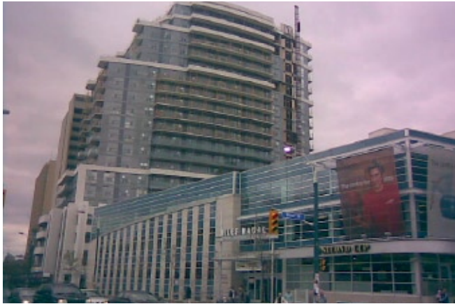
Recent development to the south of Miles Nadal JCC
