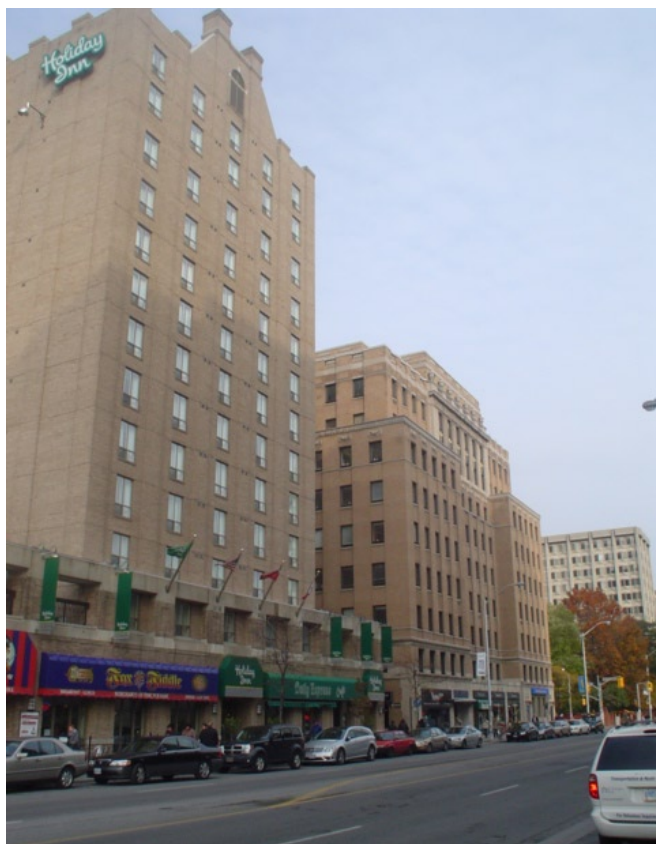
Articulation of building elements - Institutional Precinct
