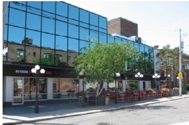
Boulevard cafe on Albany Avenue
