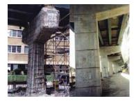
Some corroded concrete columns have been repaired.
