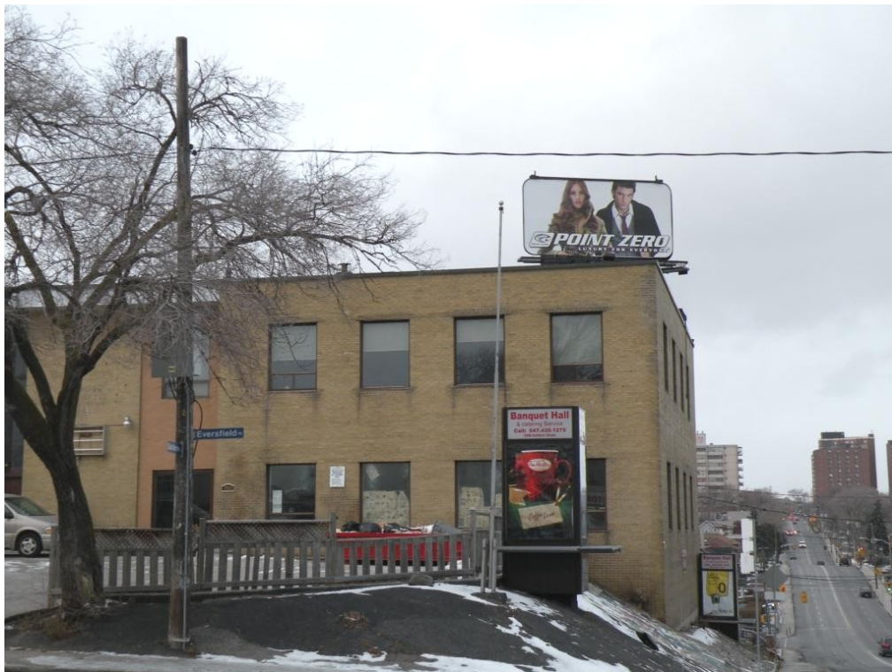
Attachment 2: Photos of the Billboard Sign at at 2080 Dufferin Street
