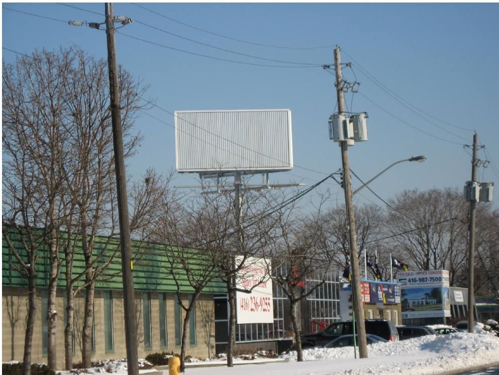
Exiting sign – East direction
