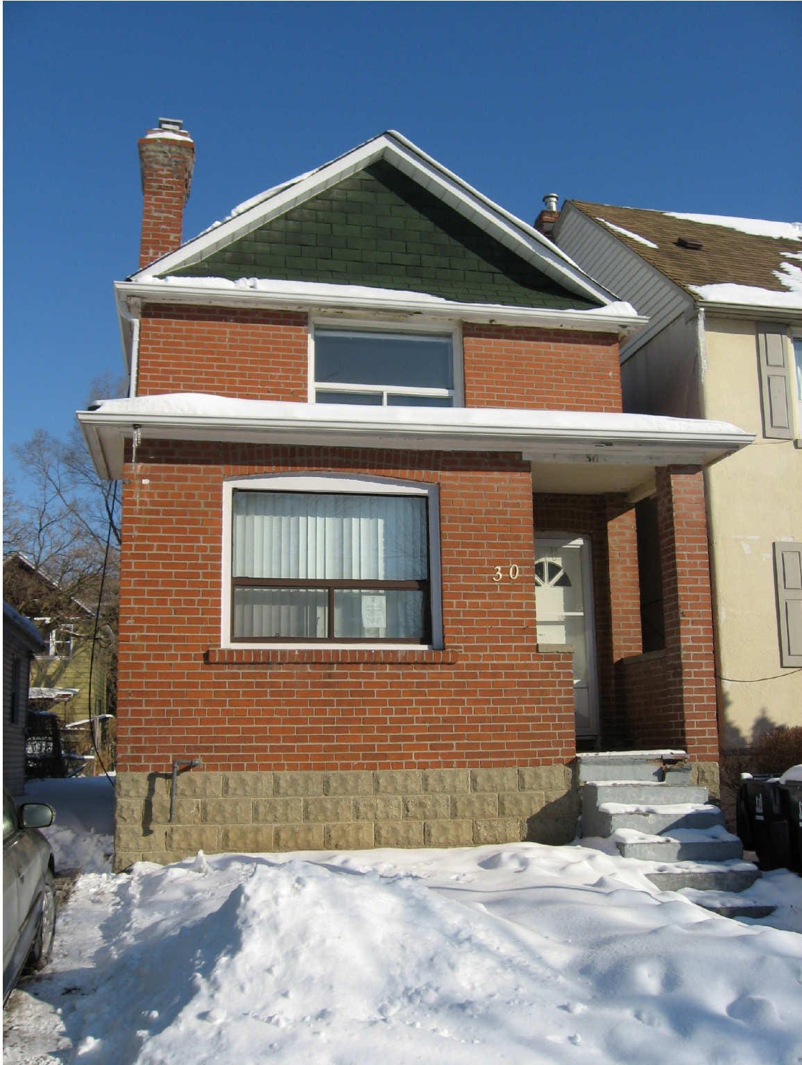
30 Warren Crescent – Front Elevation
