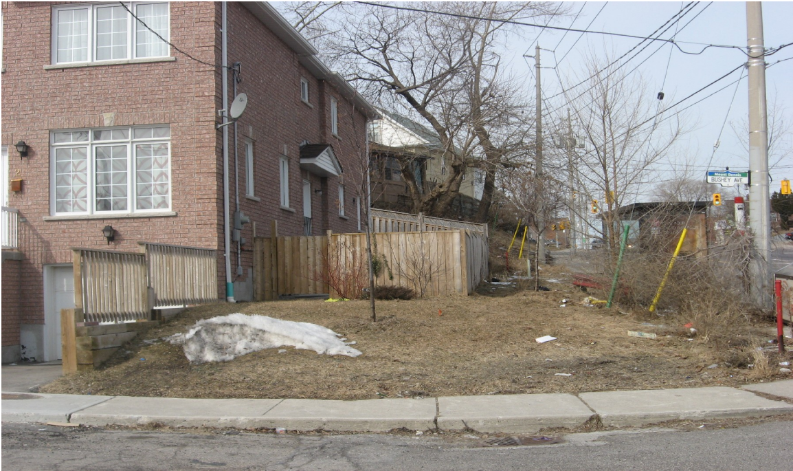
Photo of Front and side elevation – 2A Bushey Avenue
