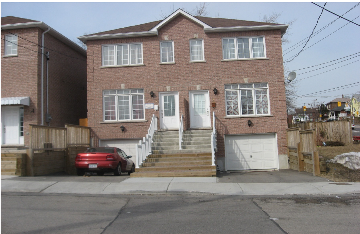
Photo of front elevation – 2A Bushey Avenue
