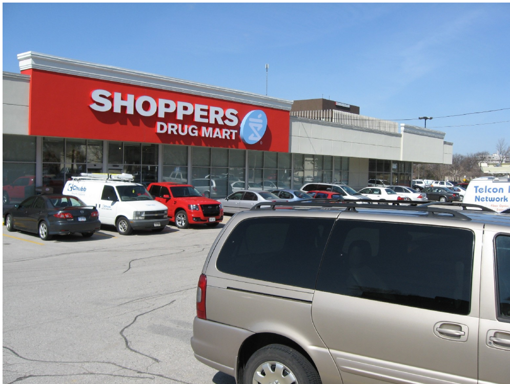
East Elevation facing The East Mall
