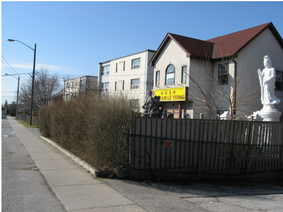
2380 Keele St that is zoned C1 and then the low rise apartments to the south of this property.
