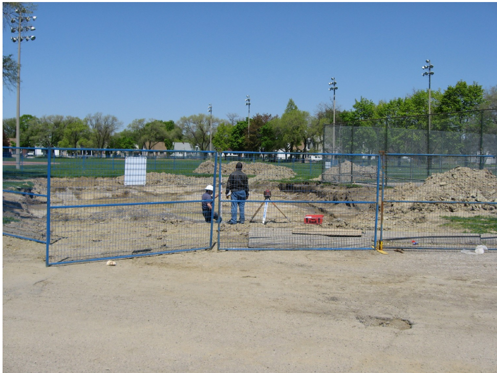
Excavation for new field house has started. Looking north from parking lot on The Queensway.
