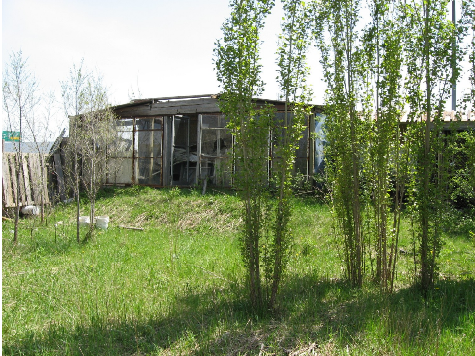
Rear yard ( behind the fence and shed is Highway 401)
