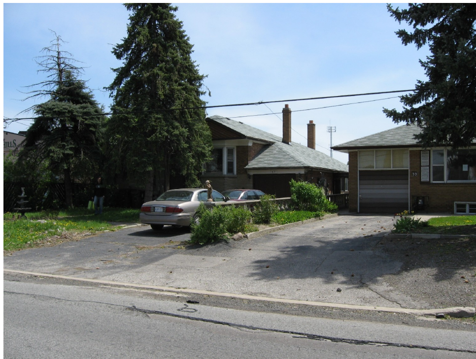
Front (north) elevation of 57 Beverly Hills Dr.
