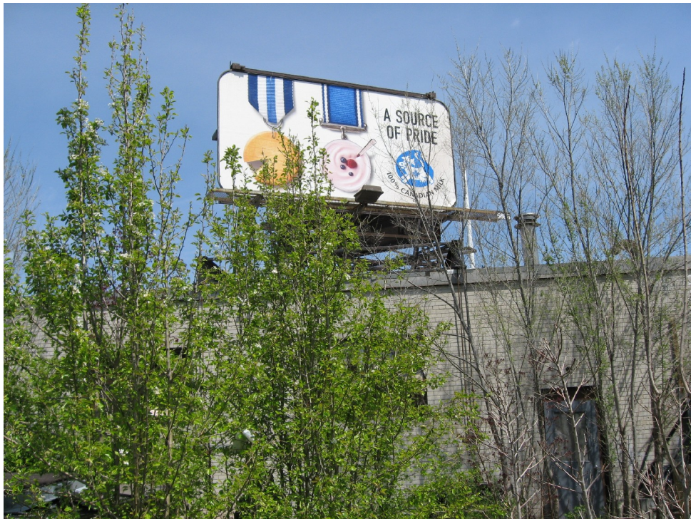
Illegal third party roof sign at 55 Beverly Hills Drive that is seen from rear yard of 57 Beverly Hills Drive the location of proposed ground sign
