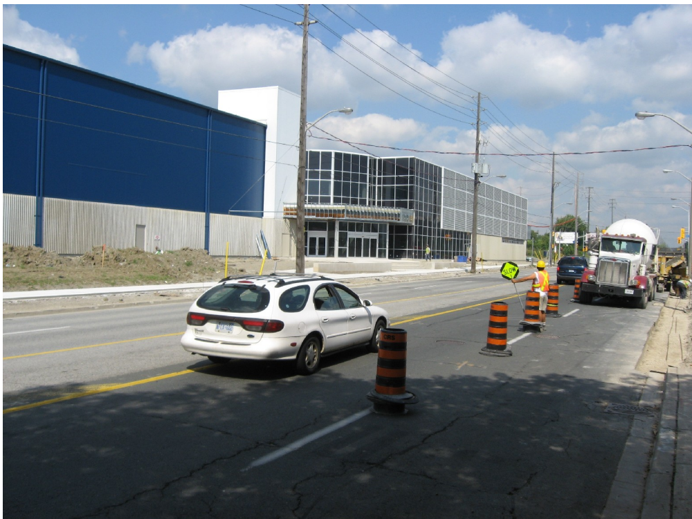
East elevation of arena looking at the main entrance off Kipling Ave
