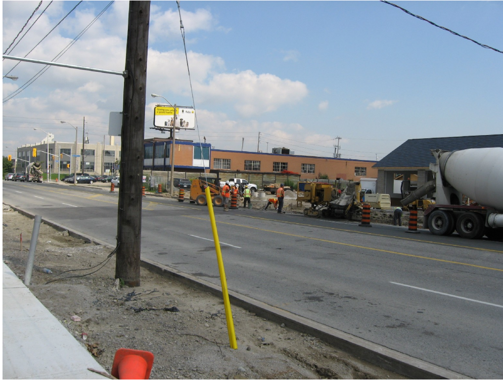
Commercial establishments on east side of Kipling Ave
