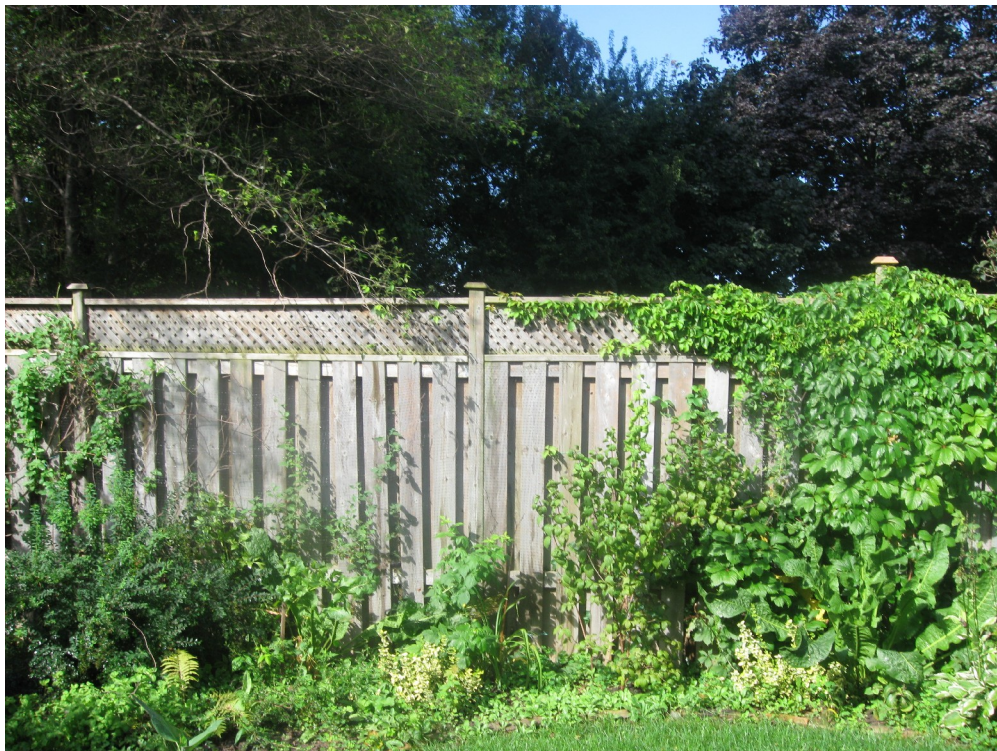
Attachment 4 - Photograph of West Elevation
