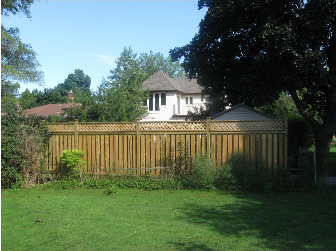
Attachment 5 - Photograph of South Elevation
