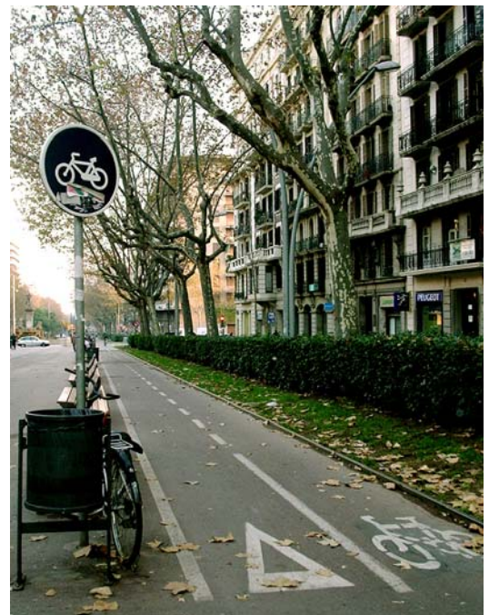
An example of an off-street bicycle trail buffered by seating and a landscaped strip with trees and bushes
