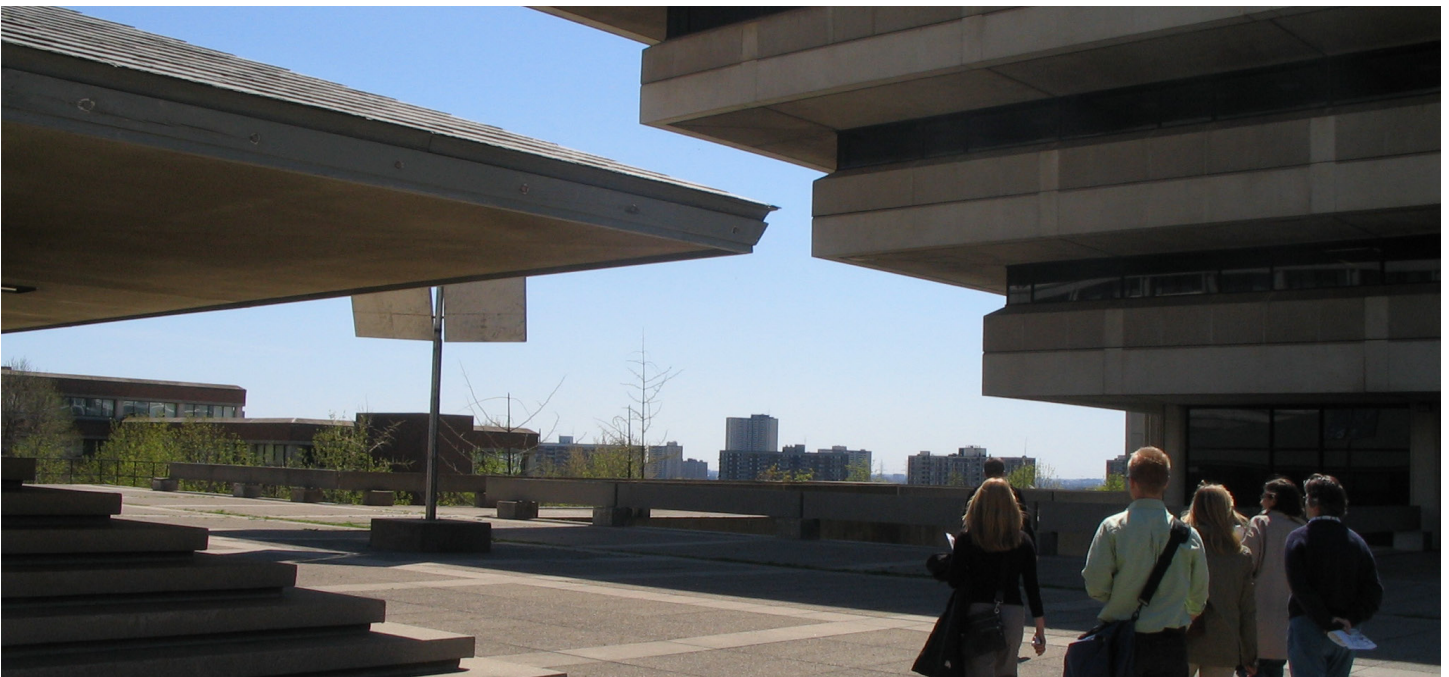
Existing York University roof terrace within the original campus buildings
