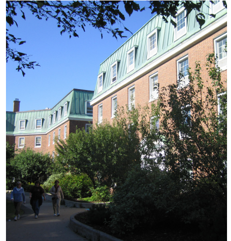
Precedent image of student residence in a courtyard style
