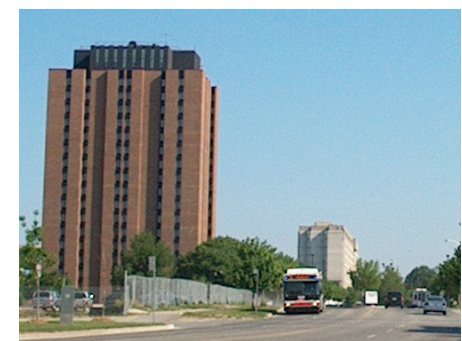
View looking north along Sentinel Road towards The Pond Road
