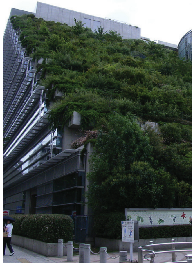
Terraced green roof design of a commercial building. Green building technologies will be encouraged on Avenue Road.
