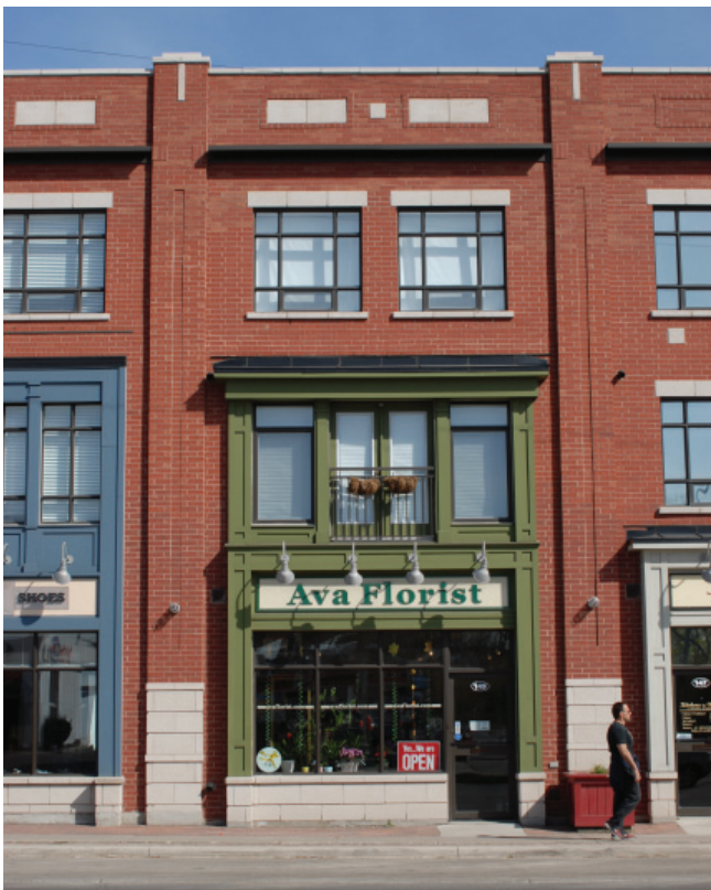
Variations in façade in the horizontal and vertical wall plane will replicate the main street character and scale.
