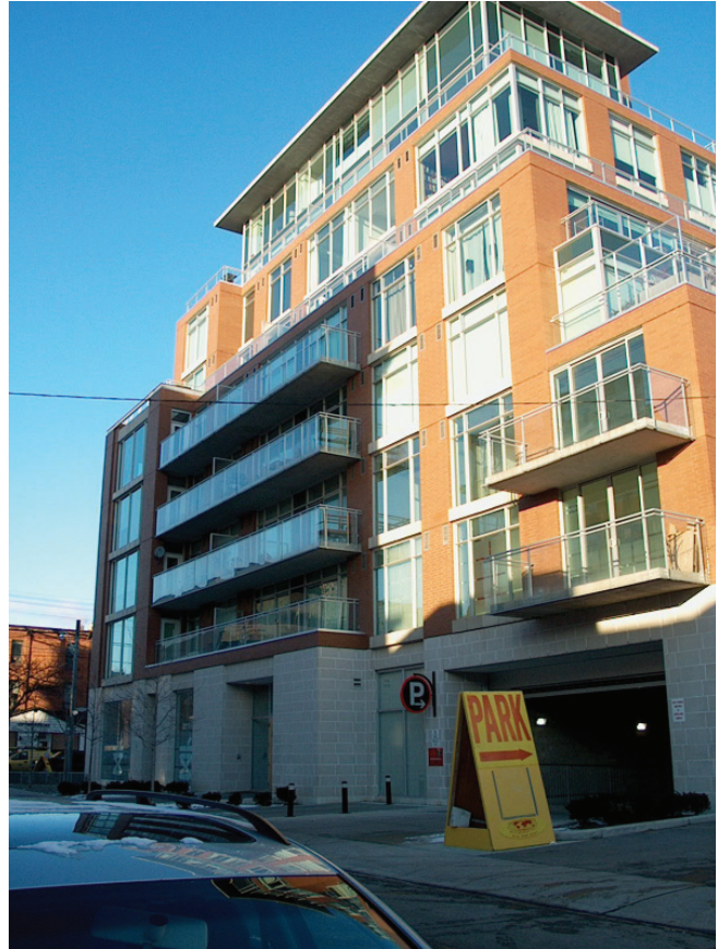
Access to below-grade parking should be located off side streets to reduce curb-cuts on Avenue Road.
