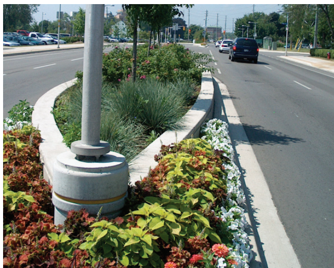
A planted median could help to improve the image of Avenue Road.
