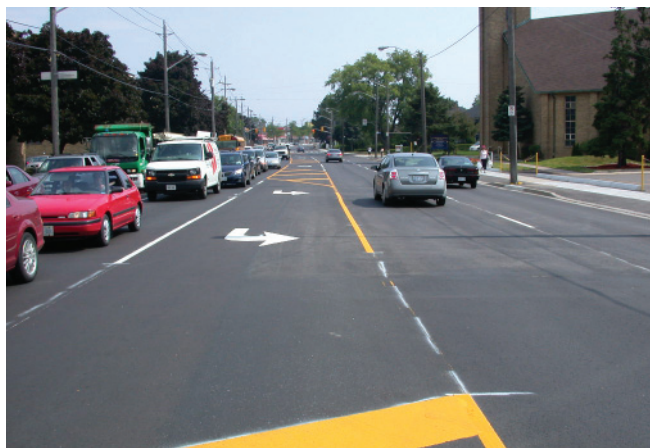
The existing painted centre median of Avenue Road.
