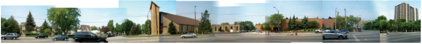
Ridley Avenue to Wilson Avenue on the west side.
